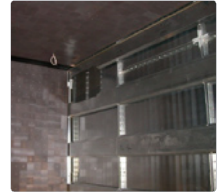
Structure for the installation of ferrite absorbers
