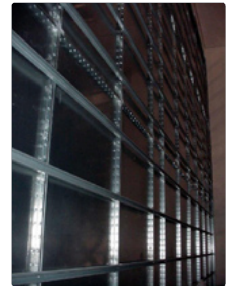
Structure for the installation of pyramid absorbers
